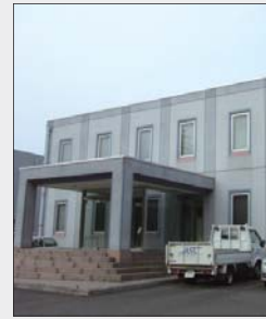
▲ ACR Aikawa Office (Aiko district, Kanagawa, Japan)
