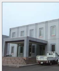
▲ ACR Aikawa Office (Aiko district, Kanagawa, Japan)
