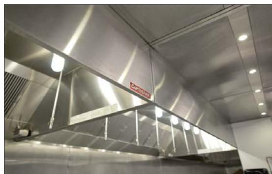
Picture 2: Sample exhaust hood system by CaptiveAire
