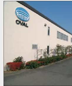
▲ OVAL Corporation Yokohama Office
