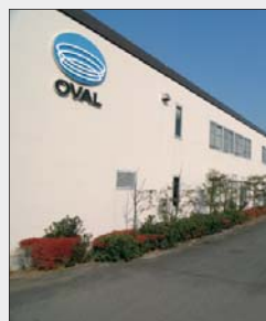
▲ OVAL Corporation Yokohama Office
